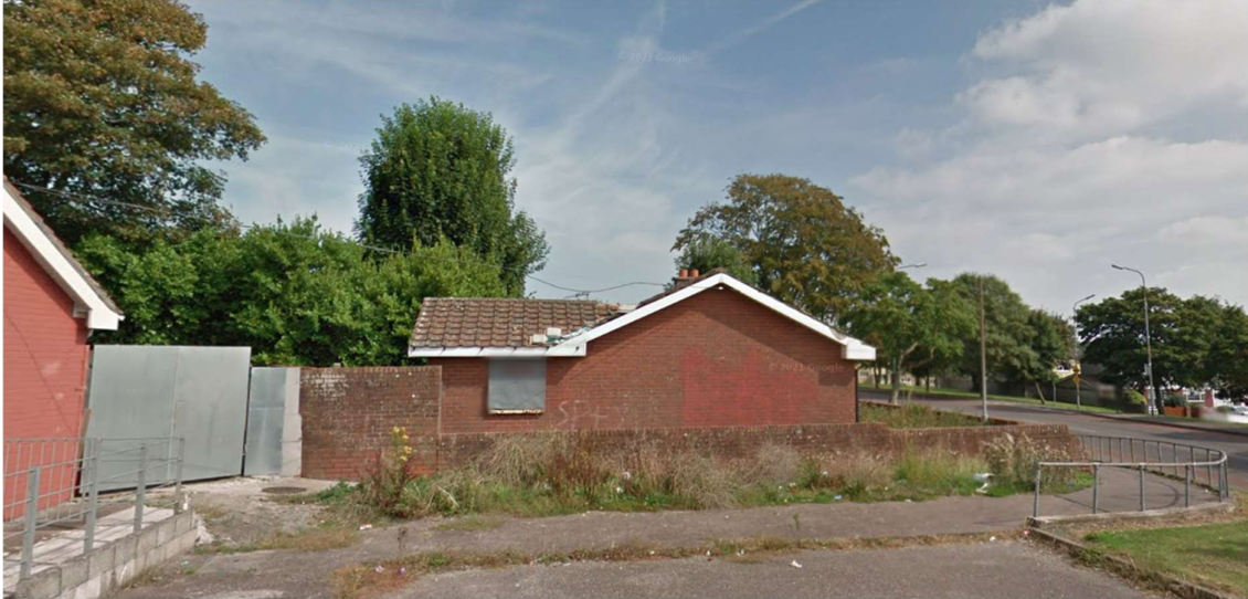
Fig. 15: Photo from 2014 of former dwellings at 101-102 now demolished.
