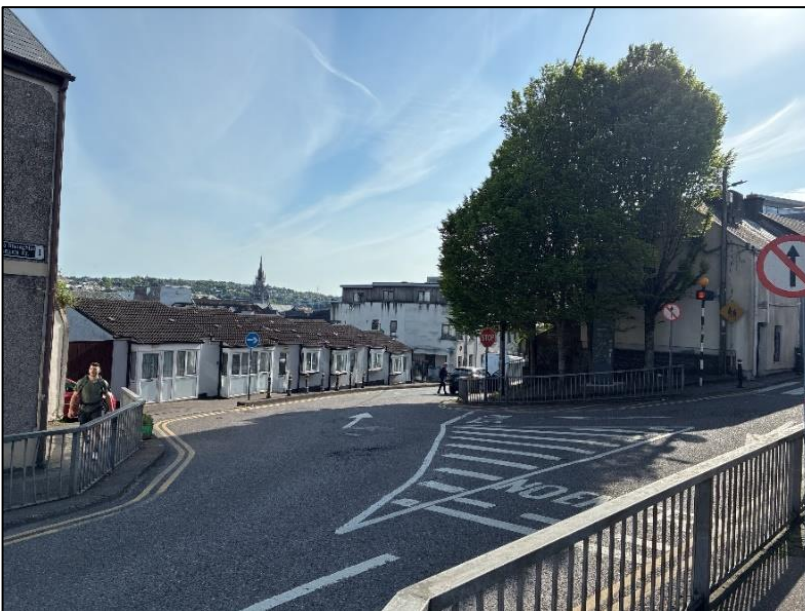
Figure 4-2 – Buildings and artificial surfaces (BL3) with scattered tree planting at the junction of Evergreen Street and Abbey Street.
