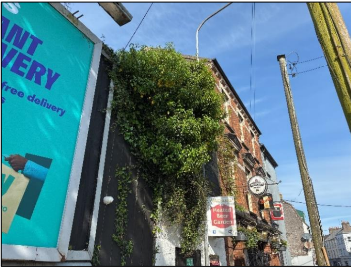
Figure 4-13 – Vegetation growth on a wooden fence bordering a private garden area on Douglas Street.
